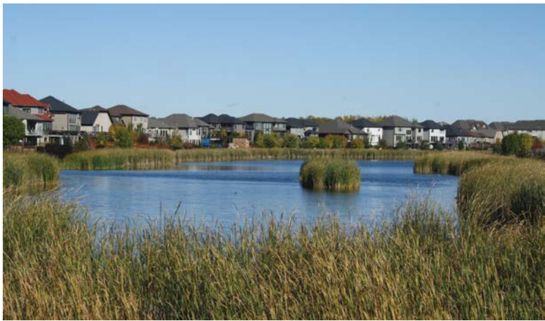
The naturalized stormwater retention pond in Winnipeg's Royalwood Phase II development. PHOTO: CHRIS PENNER
